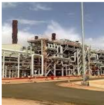
IN AMENAS COMPRESSION PROJECT
