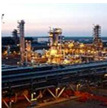
KASHAGAN EP OFFSHORE PROJECT
