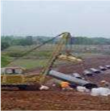
BOTAS NATURAL GAS LOOP LINES PROJECT
