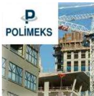
STADIUM HOTEL BY POLIMEKS CONSTRUCTION
