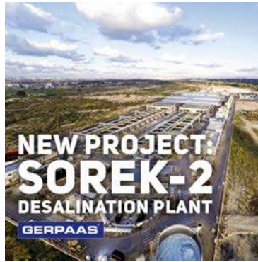
SOREK-2 DESALINATION PLANT
