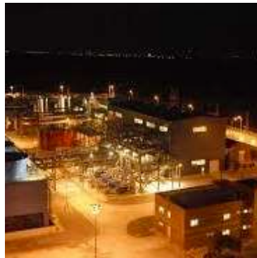
SIEMENS GERMENCIK GEOTHERMAL POWER PLANT PROJECT
