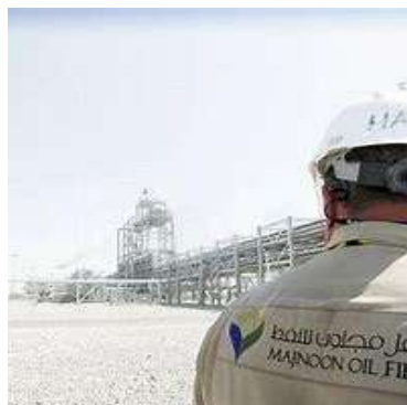
MAJNOON132/33KV GRID SUBSTATION BASRA OIL COMPANY (BOC)
