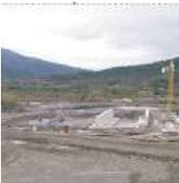
TASOVA HYDRO ELECTRICAL POWER PLANT PROJECT
