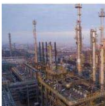
AMMONIA PLANT IN UZBEKISTAN FOR MHI
