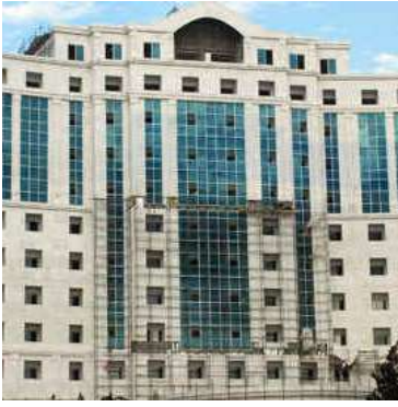
SEHIL CONSTRUCTION TURKMENISTAN PROJECTS
