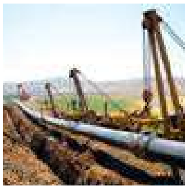
BOTAS BOZOYUK-SECKOY NATURAL GAS LOOP LINES
