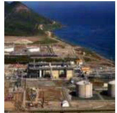
ENKA CONSTRUCTION, SAKHALIN1 PROJECT
