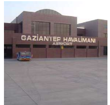
GAZIANTEP AIRPORT PROJECT
