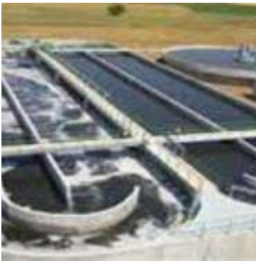
IZSU KEMALPASAWASTE WATER TREATMENT PLANT PROJECT
