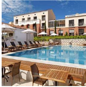
ALACATI HOTEL, ANT CONSTRUCTION
