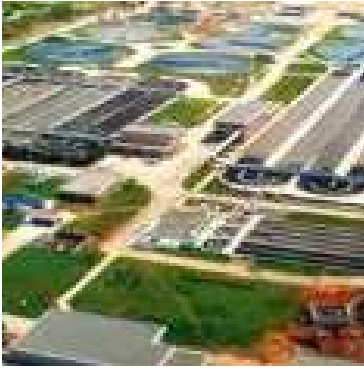
AFYON SUHUT WASTE WATER TREATMENT PLANT
