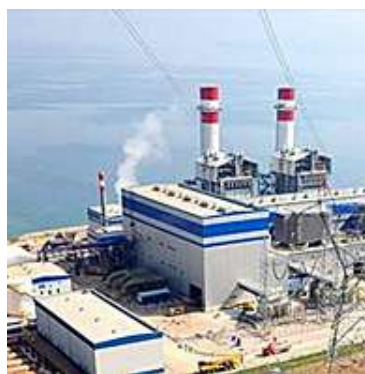
ABB AG, GES, CCPP BANDIRMA PROJECT
