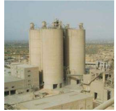
ZLETEN CEMENT PLANT PROJECT
