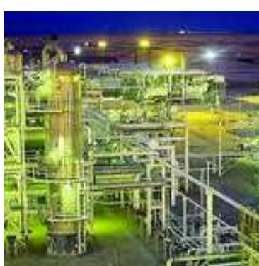
SAIH RAWL CENTRAL PROCESSING PLANT (SRCPP)
