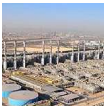
RASLANUFNEW DESALINATION PLANT, SIDEM
