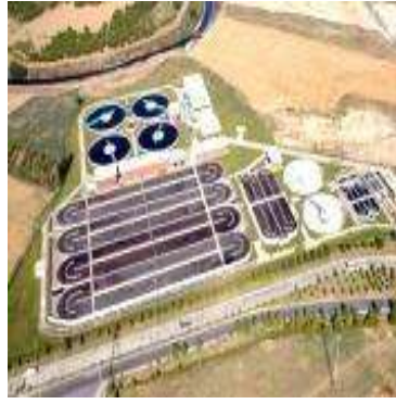
DOSAB WATER TREATMENT PROJECT
