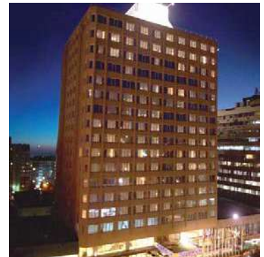
DEDEMAN HOTEL RENOVATION PROJECT
