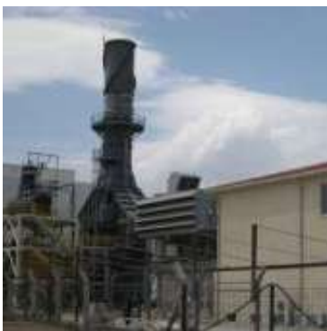
UGUR ENERGY ELECTRICAL PLANT
