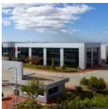
MAPACLUTCH PLANT RENOVATION PROJECT
